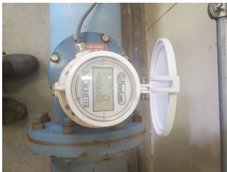
Photo 4. Master Flow Meter for Booster Pump Station
